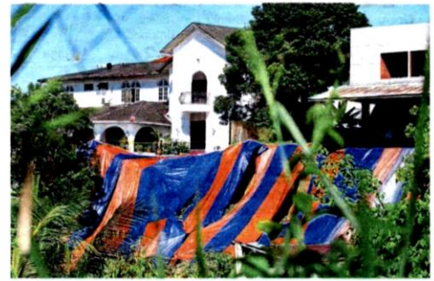
The landslide in Jalan Kemensah Heights affected three bungalows and 12 townhouses. — MUHAMAD SHAHRIL ROSLI/The Star
